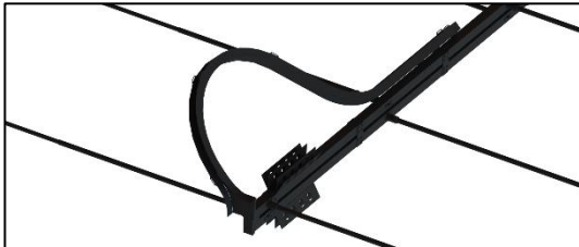
Close up view of cable management
